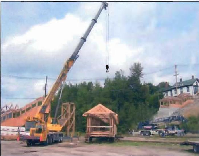
It was at that time that Robert Desrochers of Desrochers Crane Service of Derby Vermont was contacted. Because of construction site congestion, it was decided that the 114' structure would be built perpendicular to the abutments.
